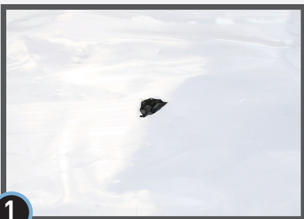
1 Occasionally, damage may cause a larger hole in the vapor barrier that requires a patch.
