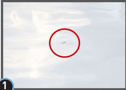
1 Small hole or slice in StegoCrawl Wrap.
