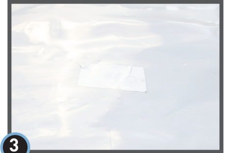
3 Center and apply StegoCrawl Tape over small hole or slice in StegoCrawl Wrap.
