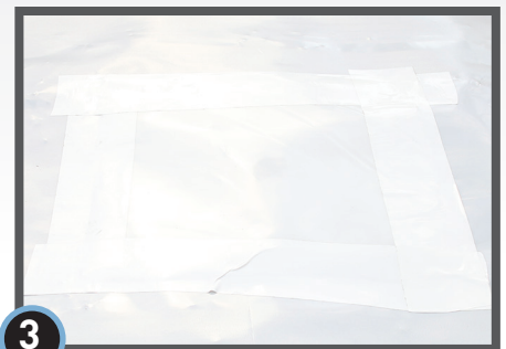
3 Seal patch with StegoCrawl Tape.
