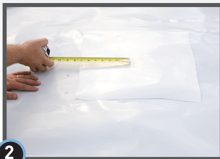
2 Clean area of adhesion. Measure and cut a piece of StegoCrawl Wrap to cover damaged area 6" in all directions. Then center the StegoCrawl Wrap patch to cover the damaged area 6" in all directions.
